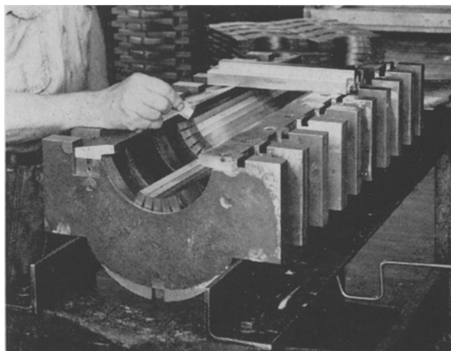
FIG. 10. Assembly of bars in barrel bar frame.
